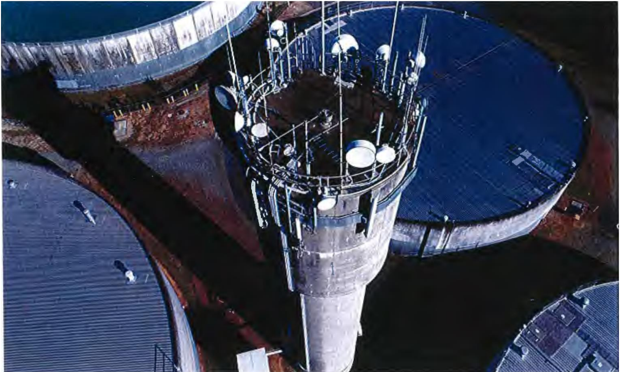
Photograph No. 1 - Aerial view of Alexandra Hills High Level Reservoir Tower
